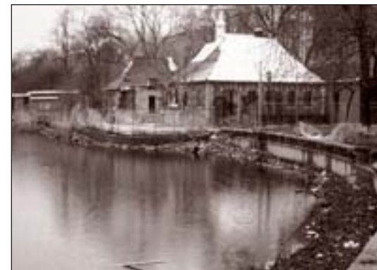
Harlem Meer Boathouse, 1980s. Notice the heavily engineered Moses shoreline bordered by silt and debris. Parts of the copper roof have been removed by vandals, and the interior has been gutted by fire.
