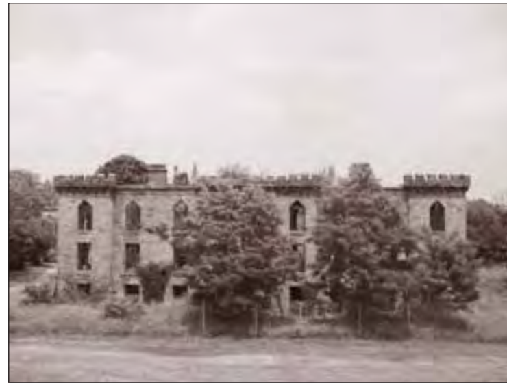
Ruins of former smallpox hospital, designed by James Renwick, Jr., 1856.
